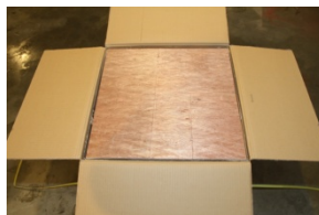
Step b, remove luan cover and place on floor
