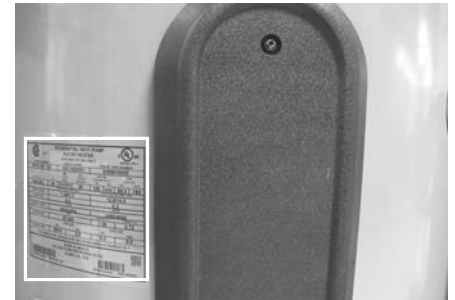
Figure 23 - The water heater’s electrical requirements can be determined from the data plate.
