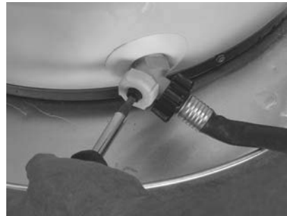
Figure 12 - Draining the old water heater.
