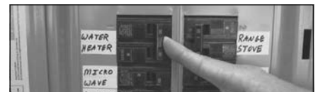
Figure 38 - Circuit Breaker
