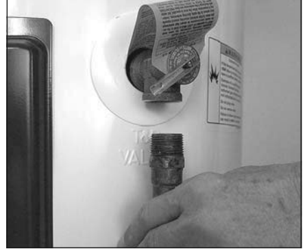
Figure 13 - Removing the T&P Relief Valve discharge pipe.
