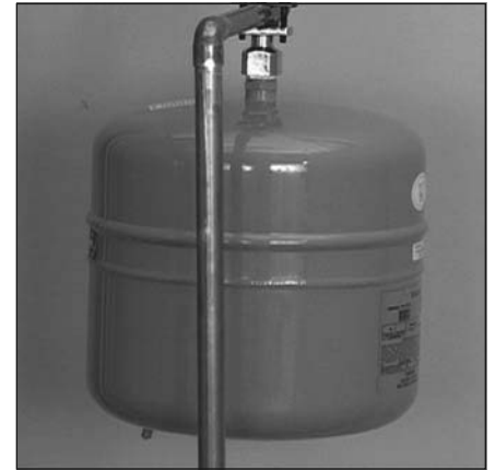
Figure 20 - The Thermal Expansion Tank should be pressurized with air, to match the home's incoming water pressure, before water pressure is applied to the tank.
