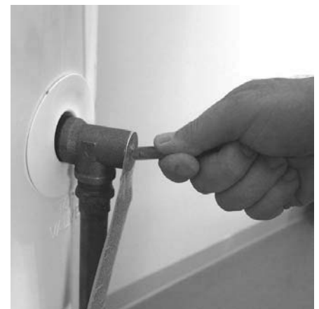
Figure 46 - T&P Relief Valve
