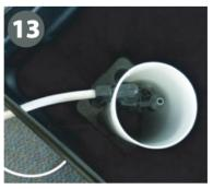
Insert hose into elbow fitting. Thread nut onto elbow hand tightened only.
