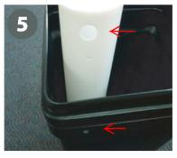
Install base and float tube into the brine tank aligning the hole in the tube with the hole in the tank.
