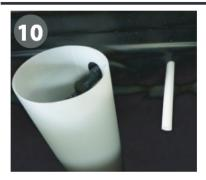
Insert hose through the hole into the brine tank.
